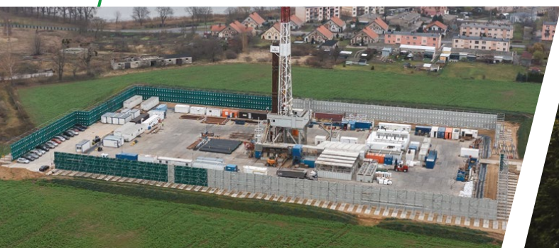
Temporary acoustic barrier with a length of 500 meters.
