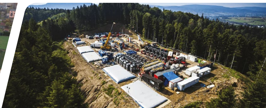
Flexible pillow tanks for water supply, storage, and transfer.
